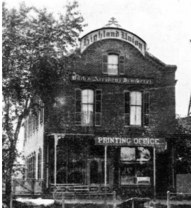
Abb. 15: Printing house of the "Highland Union", a German-language newspaper. Facade sign under the gable: „Buch und Accident Druckerei“. 12
